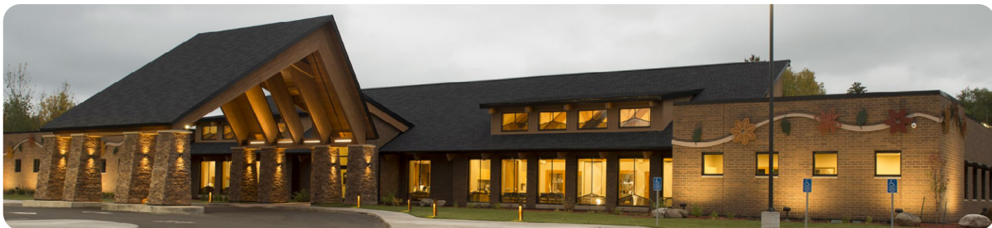
Red Cliff Community Health Center future microgrid site location
