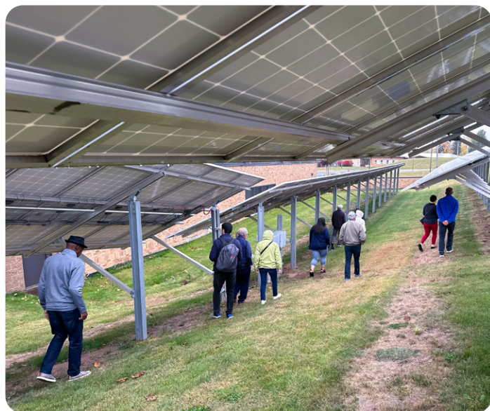
Walking tour of Bayfield County courthouse microgrid
